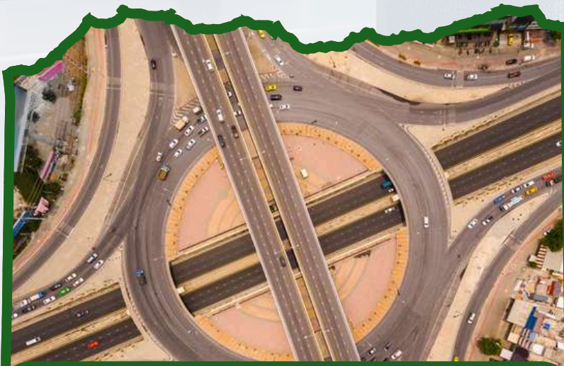
250M Express Highway Ahmedabad - Dholera
